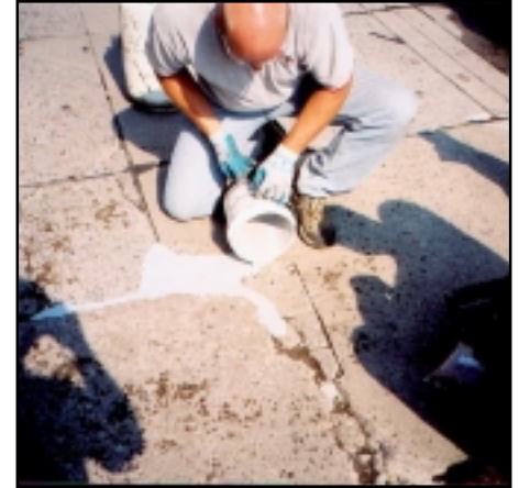
Placing special polymer patching material in larger voids
