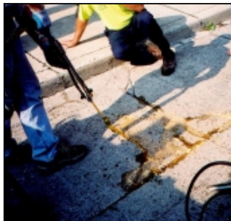
Dispensing the polymer into the cracks
